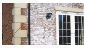
The first 3 to 5 days after laying (dependent on season), brickwork is most vulnerable to the elements as mortar is still undergoing the hardening process. Newly erected masonry should be covered by waterproof sheeting to protect fresh mortar and open cavities to stop masonry becoming saturated. Hessian is not waterproof. Once the structure is watertight, i.e. roof and windows in place, the building can commence the drying process.
